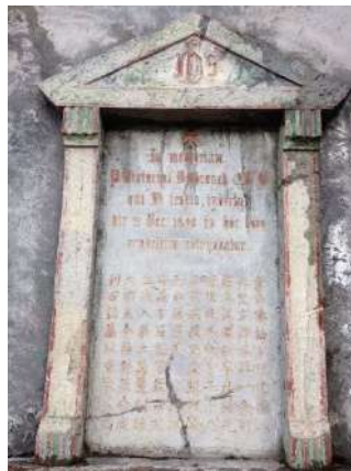
The monument stele of Fr. Delbrouck in Xiaotang. The stele was demolished during the Cultural Revolution. It was found when the church was repaired in 2019, and rebuilt here.
