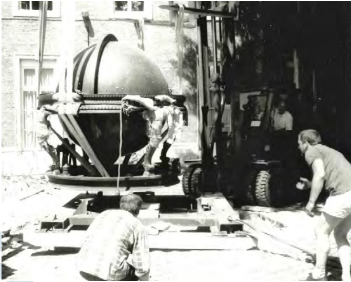
Installing the Globe at the Atrachtcollege
